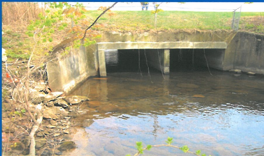
Twin Box Culverts
