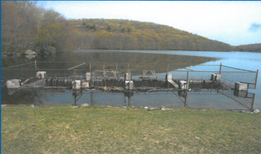
Drop Inlet Spillway
