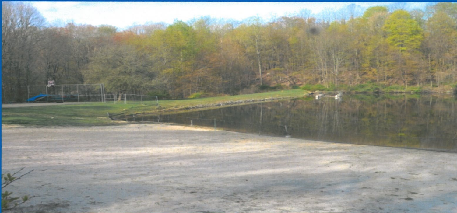
Upstream View of Dam
